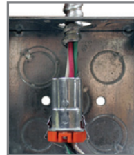
Pull conduit through knockout, insert wires in fitting
